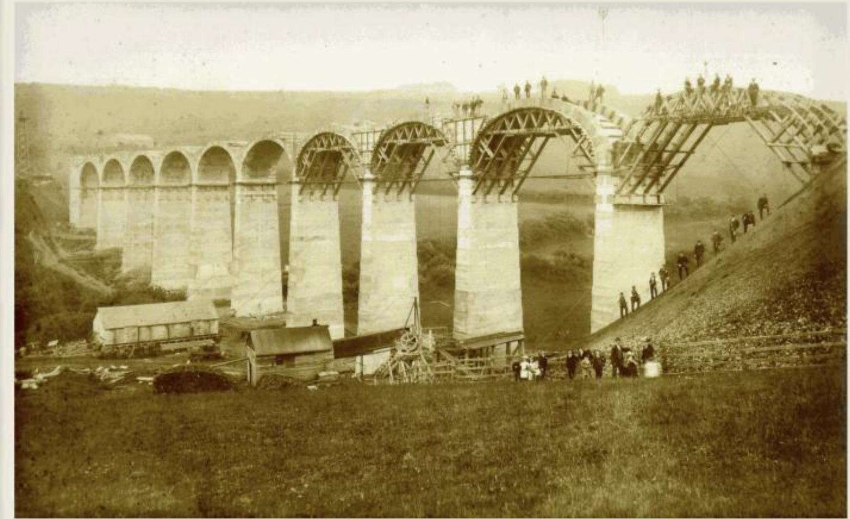
Construction of Cannington Viaduct c.1902
